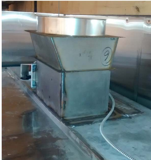
Figure 18 Closer View of Zoneflow and J-Couple with Starter piece
