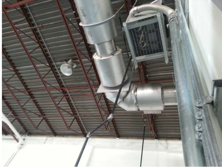
Figure 48 Adjustable Expansion Section with Horizontal Support Plate
