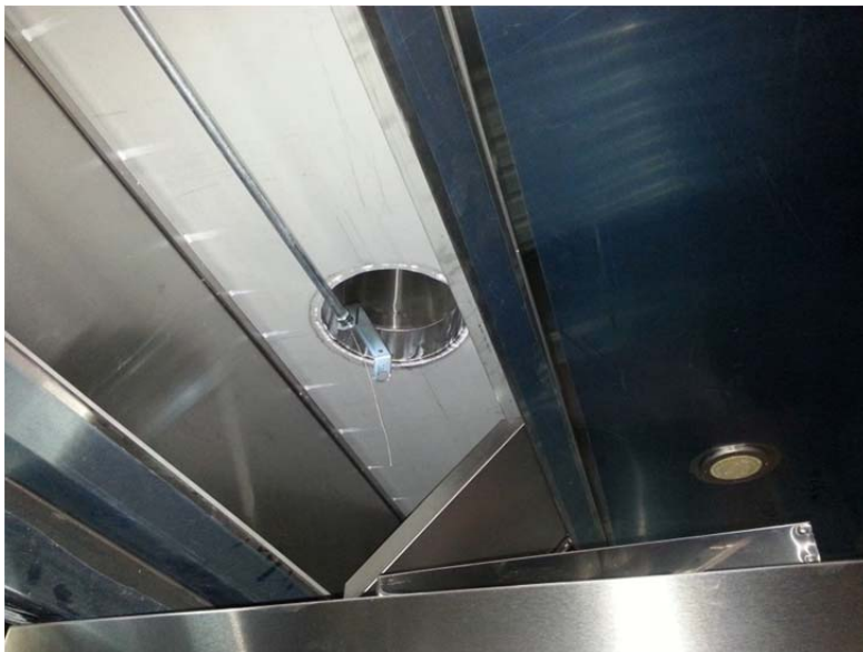
Figure 16 Looking inside a hood at welded starter section
