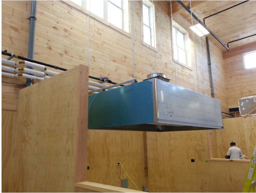
Figure 17 Spring Air FN Hood, with Zoneflow and J-Couple and Starter Piece
