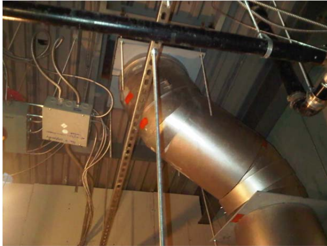
Figure 10 Offset using 30 degree elbows with no Cleanout
