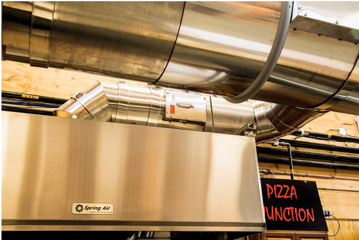
Figure 1 Spring Air FN-B-MB with Van Packer Pre-Engineered Ductwork
