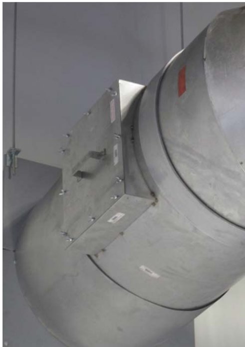
Figure 9 Cleanout on Horizontal GZ duct
