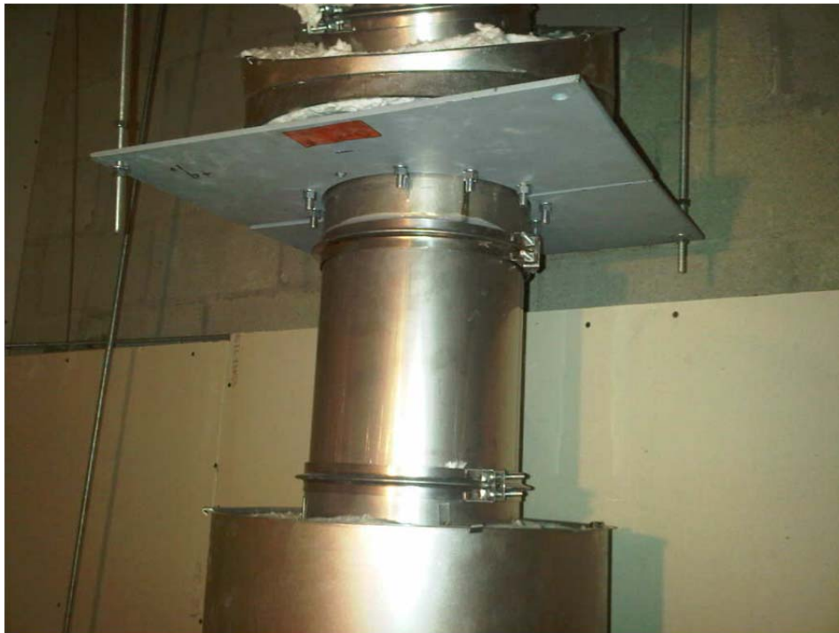
Figure 49 Vertical Support Plate under offset
