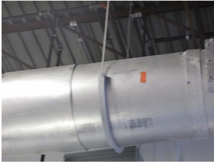
Figure 8 Horizontal GZ duct breaching
