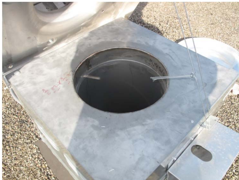
Figure 11 Spun Aluminum fan curb connection with GZ duct
